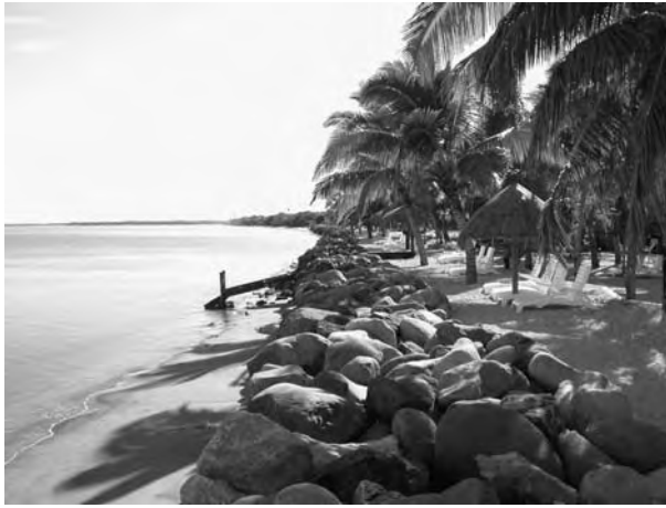
Figure 9.8 Seawall to protect the (artificial) beach and tourist accommodation at a tourist resort
