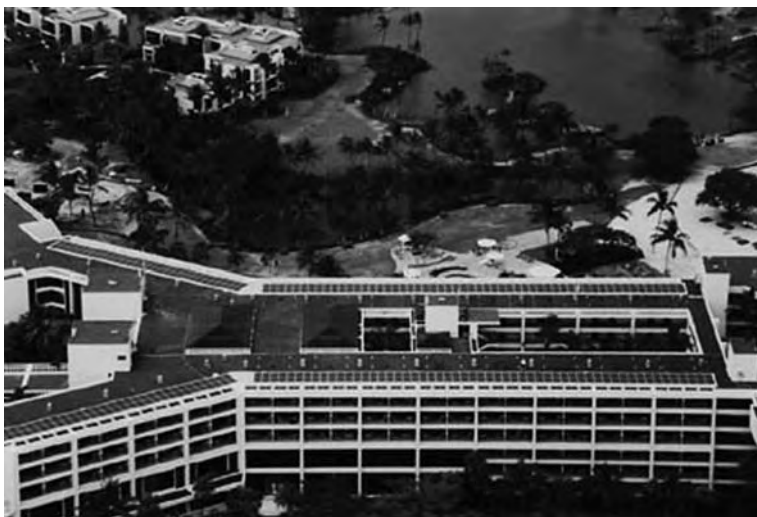
Figure 7.9 Solar panels at the Mauna Lani Bay Resort, Hawaii. The PV system supplies 674 kW of electric power, which makes Mauna Lani the largest solar-powered resort in the world.
